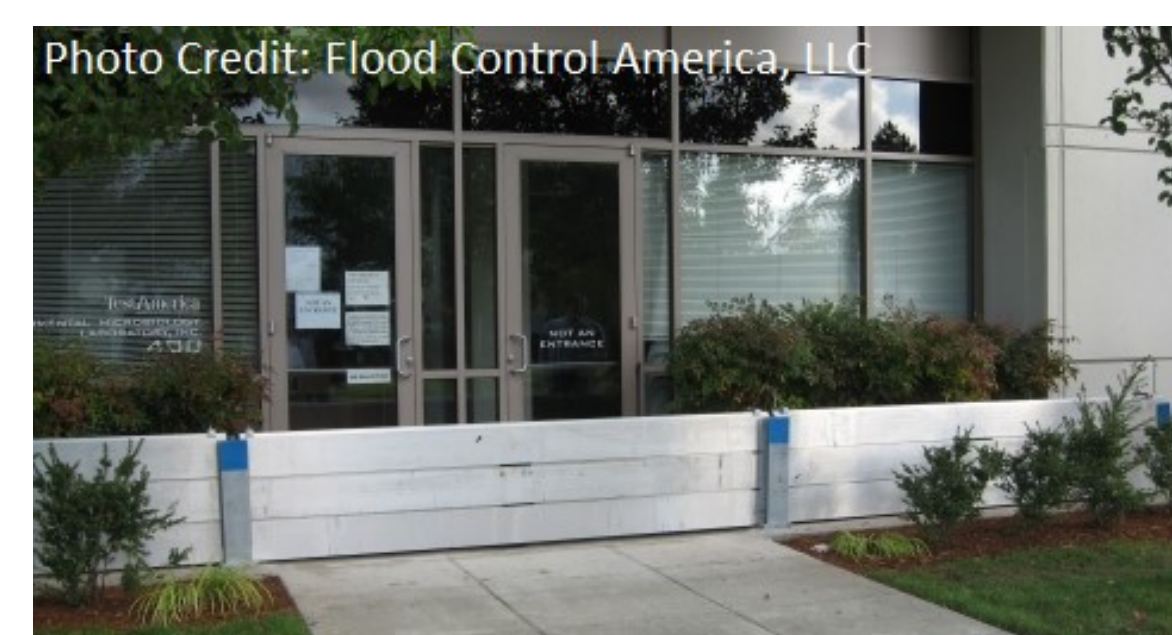
Removable flood barriers of an office, Bothell, Washington
