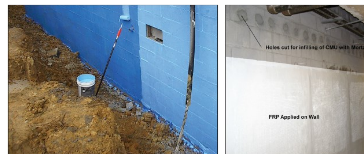
Application of waterproof membrane on exterior wall (left) and fiber-reinforced polymer wrap applied to interior wall (right)
